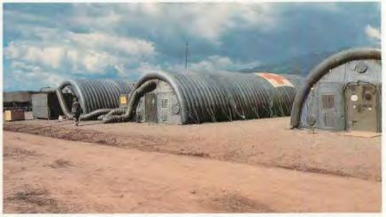
ABOVE: Inflatable MASH hospital takes six turbines burning chopper gas to keep it up.
